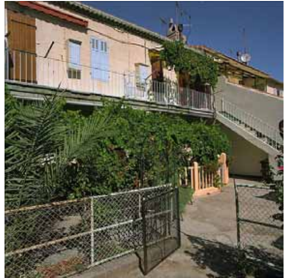
Appartment building from 1914 : frontage on court with external stairs and gangway serving the accommodations upstairs – picture M. Heller
